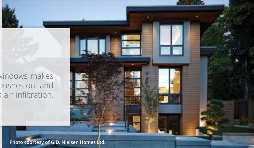
Photo courtesy of G.D. Nielsen Homes Ltd.
