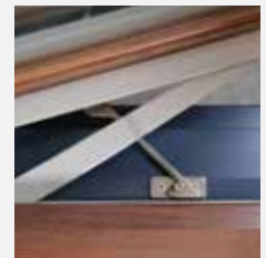
Crank-out Casement with WOCD
