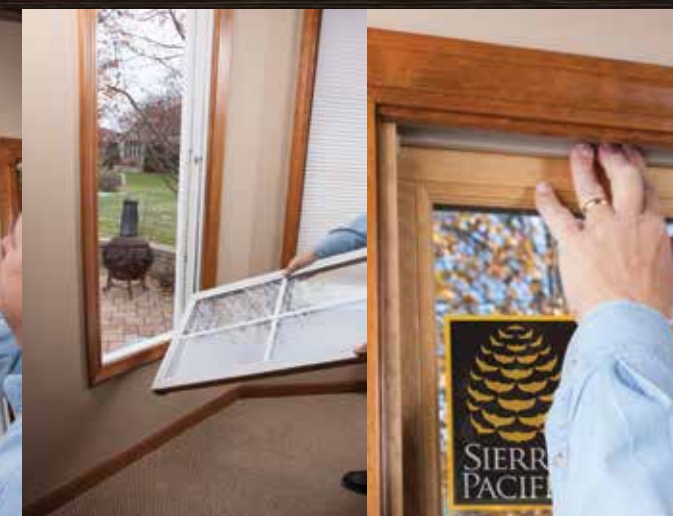
Step 3 Install new sash.
